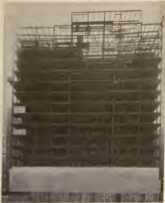
CONSTRUCTION VIEW, OLD COLONY LIFE BUILDING, CHICAGO, ILL.
